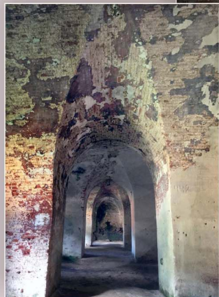
Cavalry casemate: Brickwork at its finest
